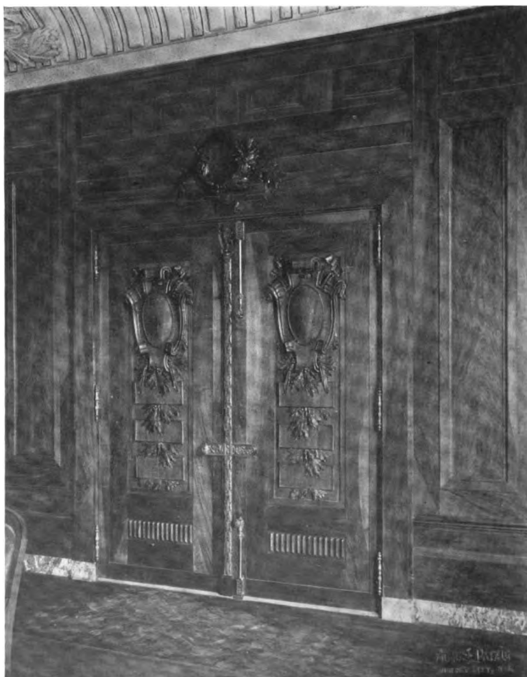
Hand Carved Doors of Circassian Walnut between Board Room and Foyer, Importers and Traders' National Bank.
